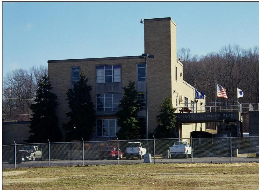
Madisonville Water Treatment Plant, Lake Peewee with supplemental intake from the Green River
